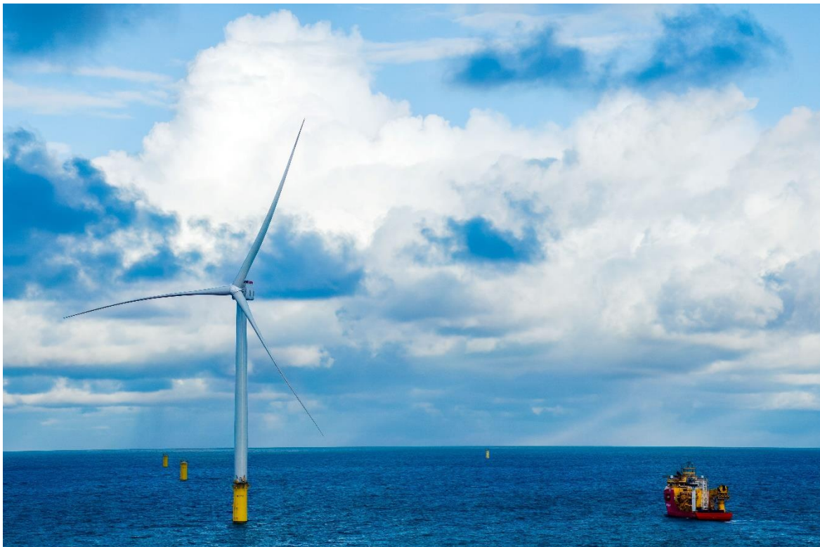
Installation works at Dogger Bank
