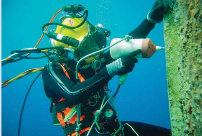
Fugro diver testing the cathodic protection of an offshore platform, Middle East.
