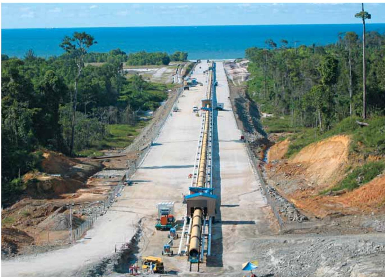
*The Gravity Actuated Pipe (GAP™) for the Kikeh field, consisting of a (yellow) carrier pipe and (white) high pressure fluid transfer lines, nearing completion at the assembly and launching site on the coast of Borneo*
