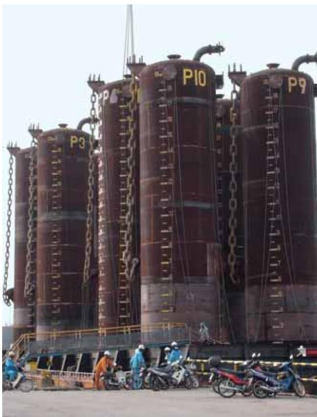
*Suction piles for the anchoring of the FPSO Kikeh to be installed by the 'Normand Installer' at a water depth of 1,350 metres*
