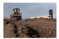
The A50 between Ewijk and Valburg is widened and the interchanges are changed dramatically. At the interchange Ewijk a completely new exit of Den Bosch to Nijmegen is developed where a lot of sand is needed. Sand is expensive, scarce and finite as a raw material. It was therefore decided to use incineration ash from the waste power plants, a secondary raw material.
