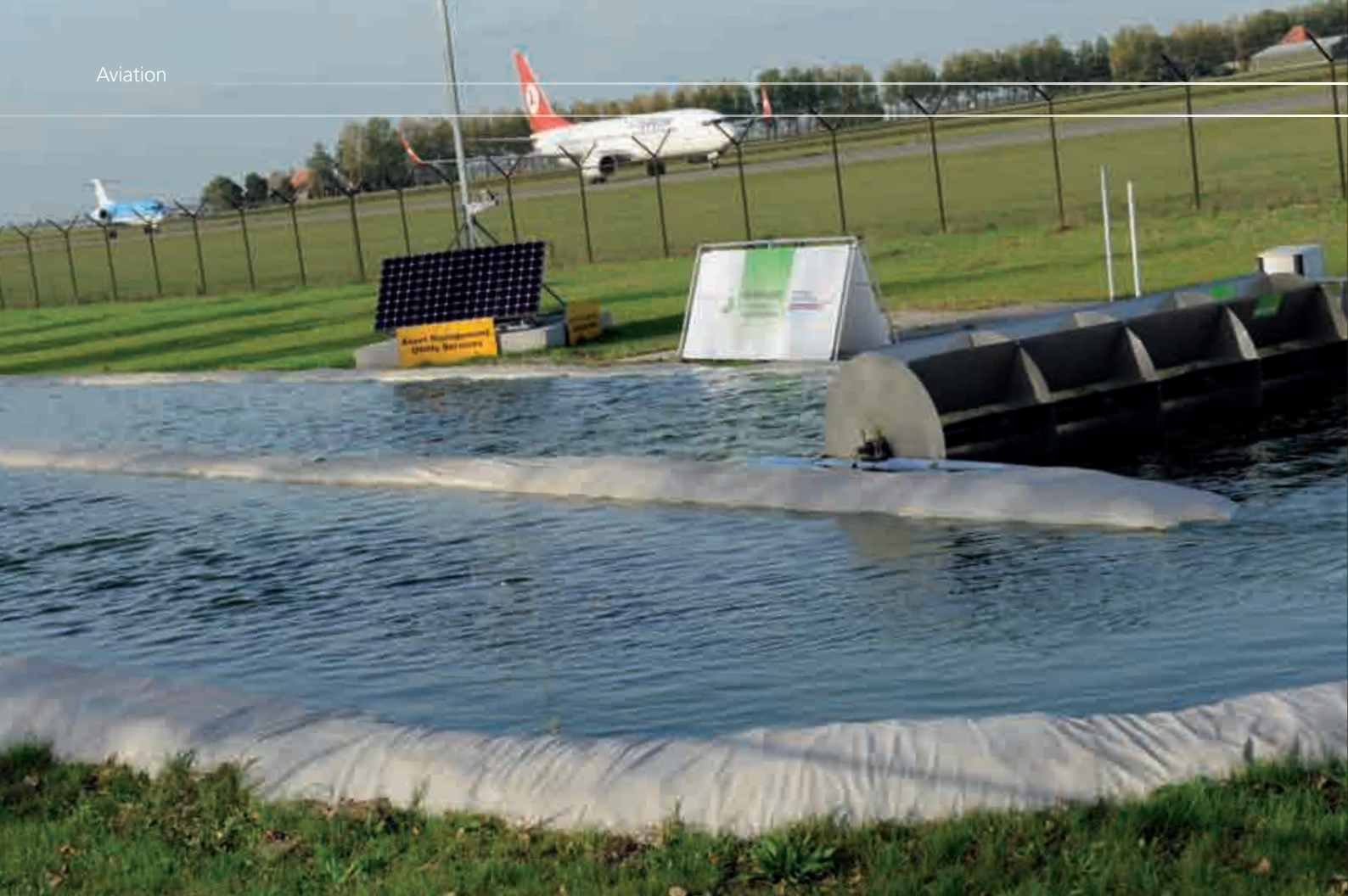
Algae basin The micro algae basin is one of the sustainable innovations started this year. The aim of the algae basin is to test whether algae can be used to break down glycol and potassium acetate in water in an environmentally friendly manner. Micro algae produce large quantities of oxygen, which breaks down glycol. The carbon dioxide released is absorbed by the micro algae and what remains is purified oxygen-rich water and algae biomass.
