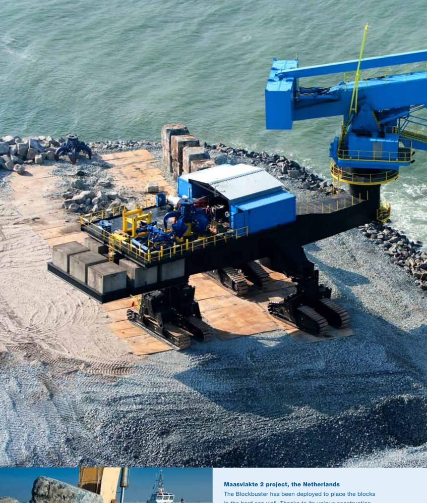
The Blockbuster has been deployed to place the blocks in the hard sea wall. Thanks to its unique construction this 'E-crane' is able to lift blocks weighing 50 tonnes and move them across a distance of 63 meters. Both the technical adjustments needed to achieve this and the advanced operating system were developed in-house by Boskalis.
