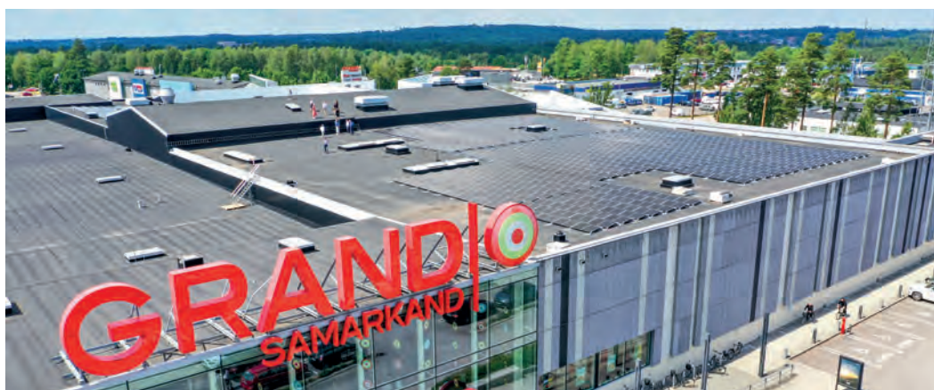
Solar panel roof installation at Grand Samarkand.
