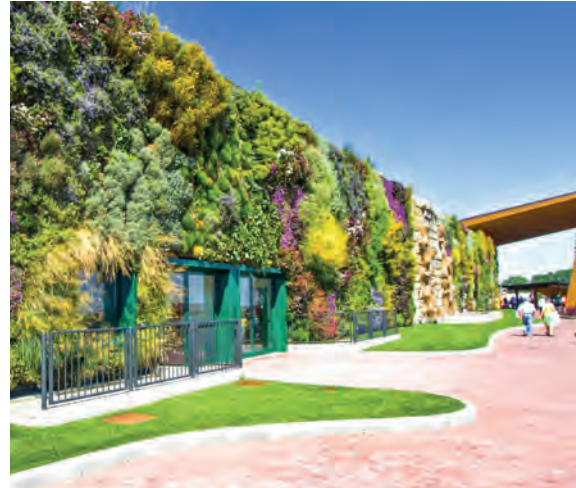
Green wall at Fiordaliso.
