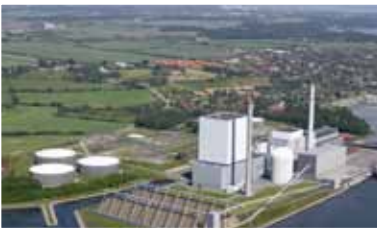
New biomass-fired power plant (DONG)
