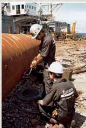
Mounting measuring tools on an offshore pile
