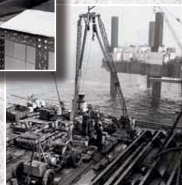
First offshore CPT at the Leman Bank
