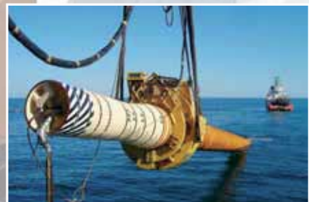
Installation of anchoring pile in the Caspian Sea
