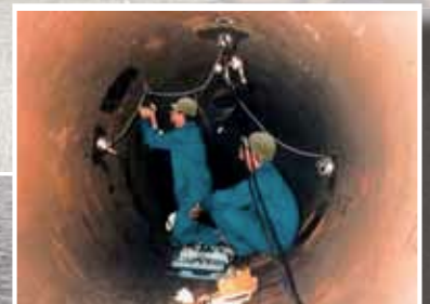
Mounting measuring equipment for monitoring driven pile
