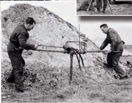
Installing ground anchors for CPT test
