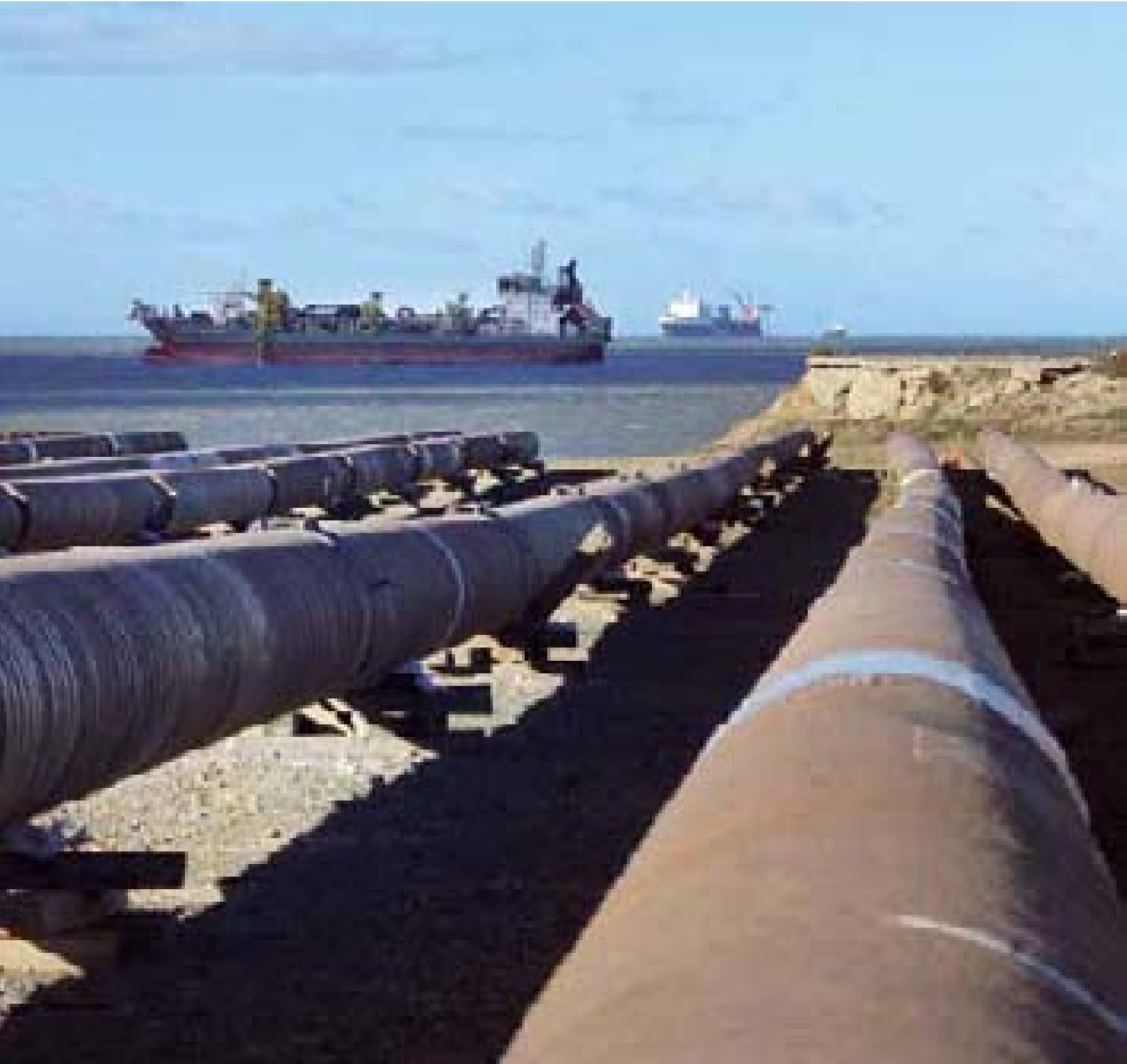
Off the southernmost point of South America, in the Magellan Strait, the trailing suction hopper dredger Prins der Nederlanden dredged a trench for the 35 kilometer gas pipeline. The area is known for its high tidal conditions, unpredictable weather and strong currents.
