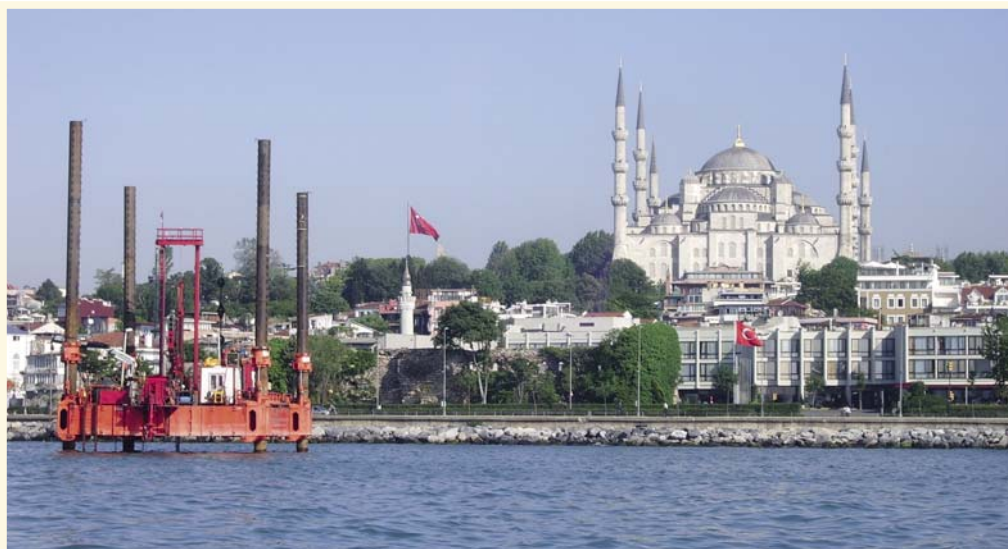
Eurasia Tunnel Project. Skate IV jack-up platform working in the Bosphorus Strait in front of the old town of Istanbul, Turkey.
