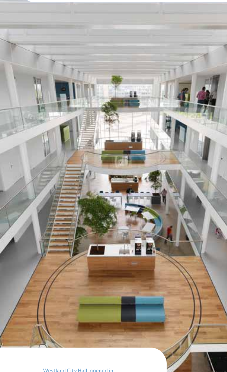
Westland City Hall, opened in September 2017
