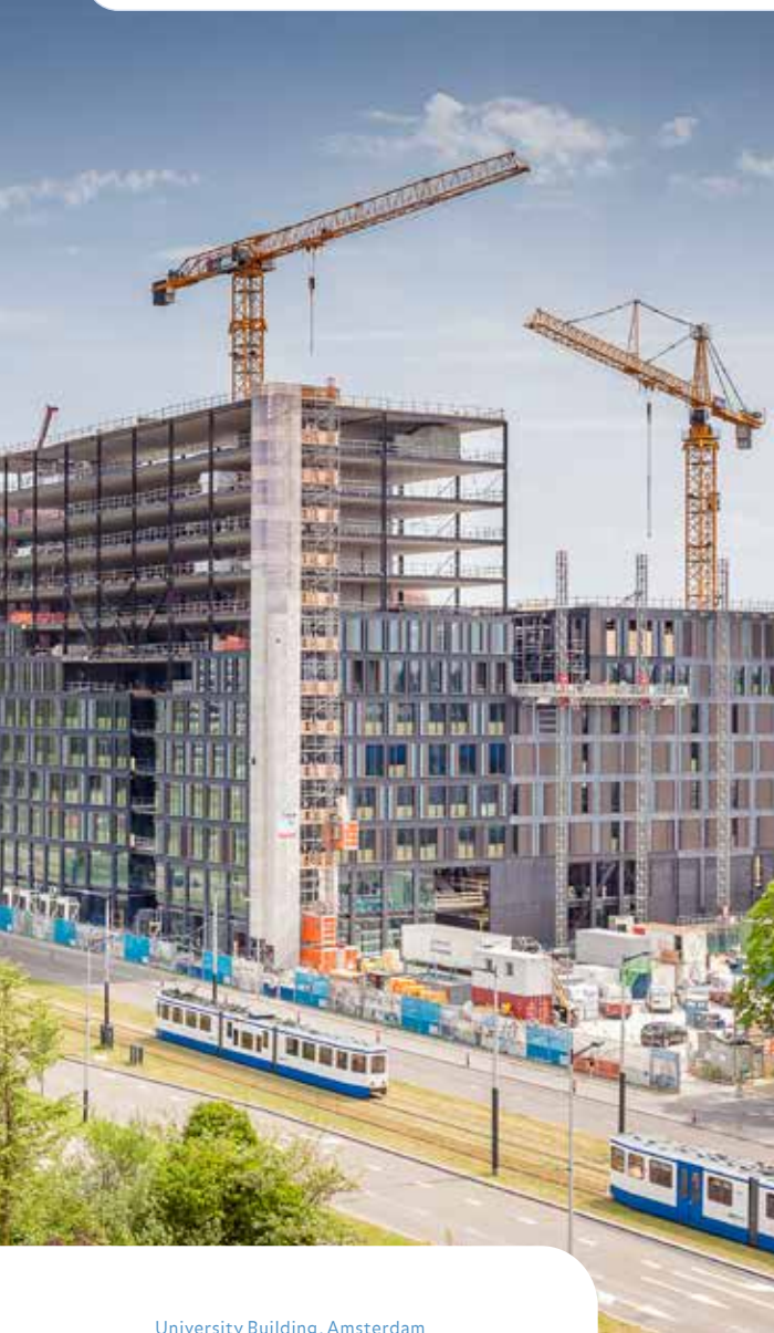
University Building, Amsterdam
