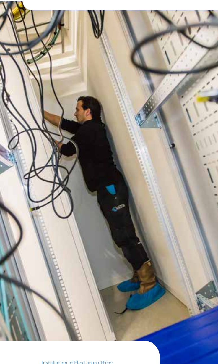
Installation of FlexLan in offices
