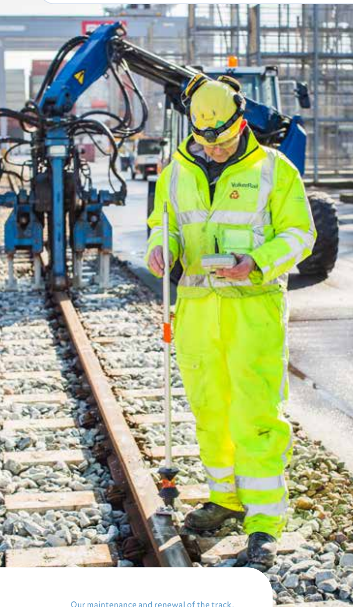
Our maintenance and renewal of the track, switches and crossings, overhead line infrastructure and signaling prevents breakdowns, delays and unsafe situations. VolkerWessels also has the people and capability to construct new sections and replace existing lines
