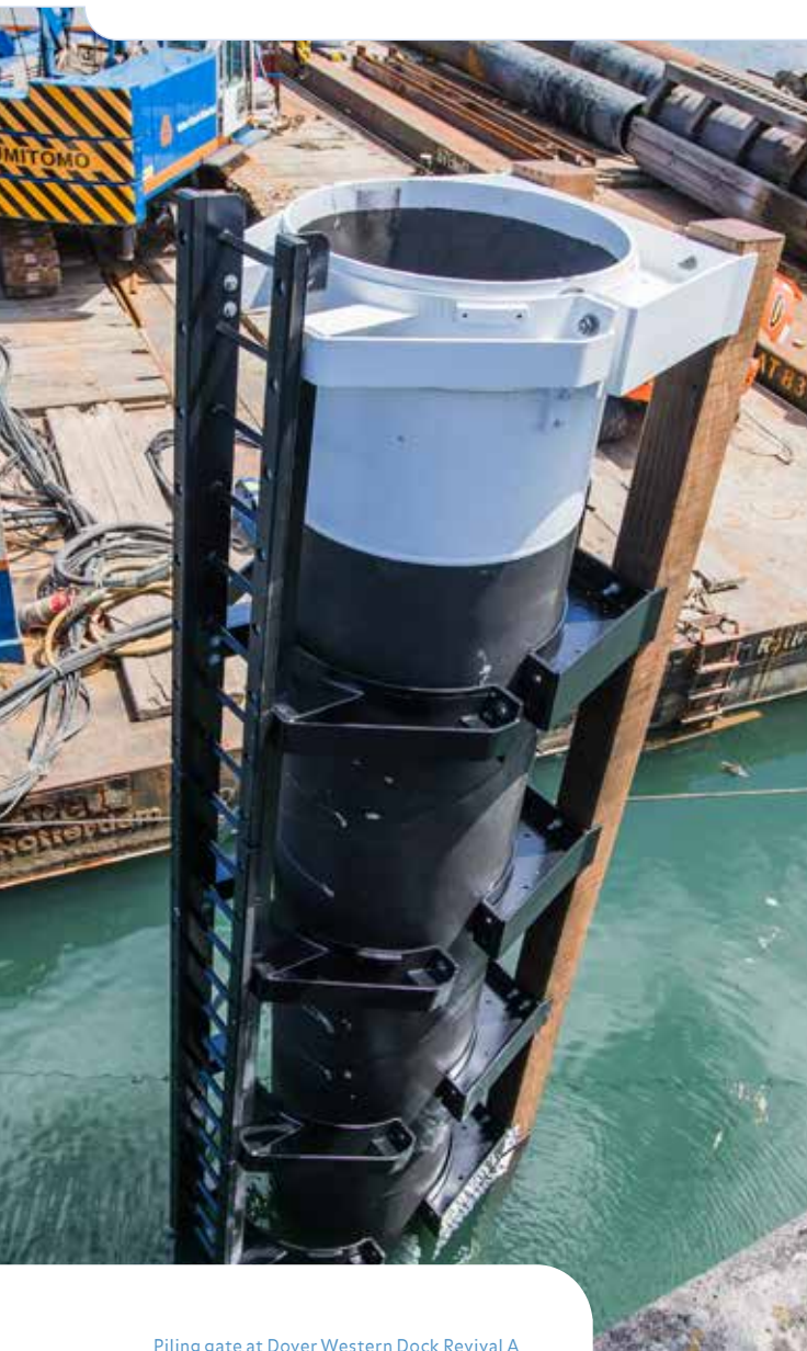
Piling gate at Dover Western Dock Revival A
