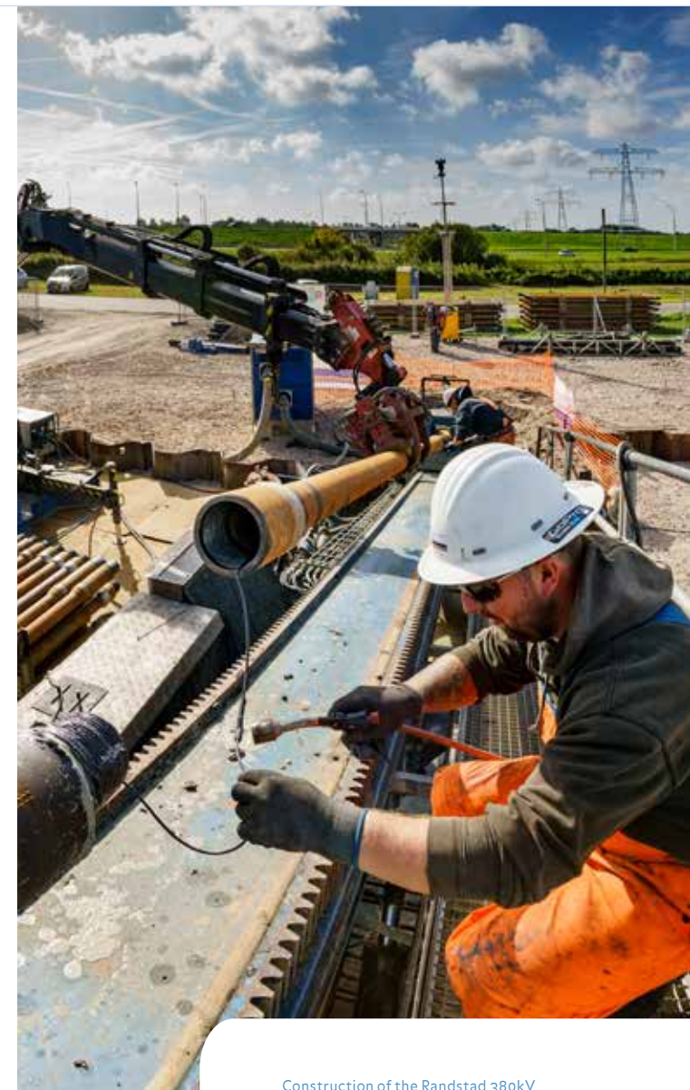
Construction of the Randstad 380kV electricity highway
