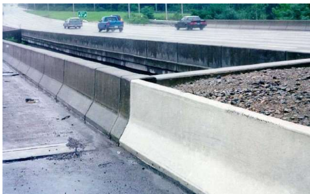
Fig. 7: Concrete road barriers based on grey and white cement, respectively, illustrating the improved visibility of white concrete under wet conditions.
