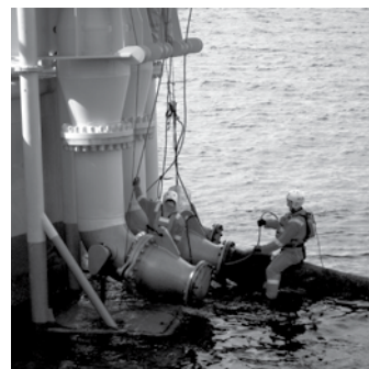
Top: Hook up operation of the marine offloading hose to a deepwater CALM buoy Bottom: SBM Offshore employee
