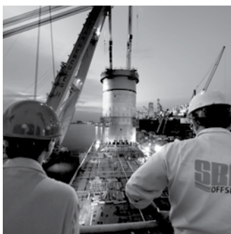
Left: Manifold section of the turret of FPSO Capixaba Right: Lifting operation of the lower section of the Skarv FPSO
