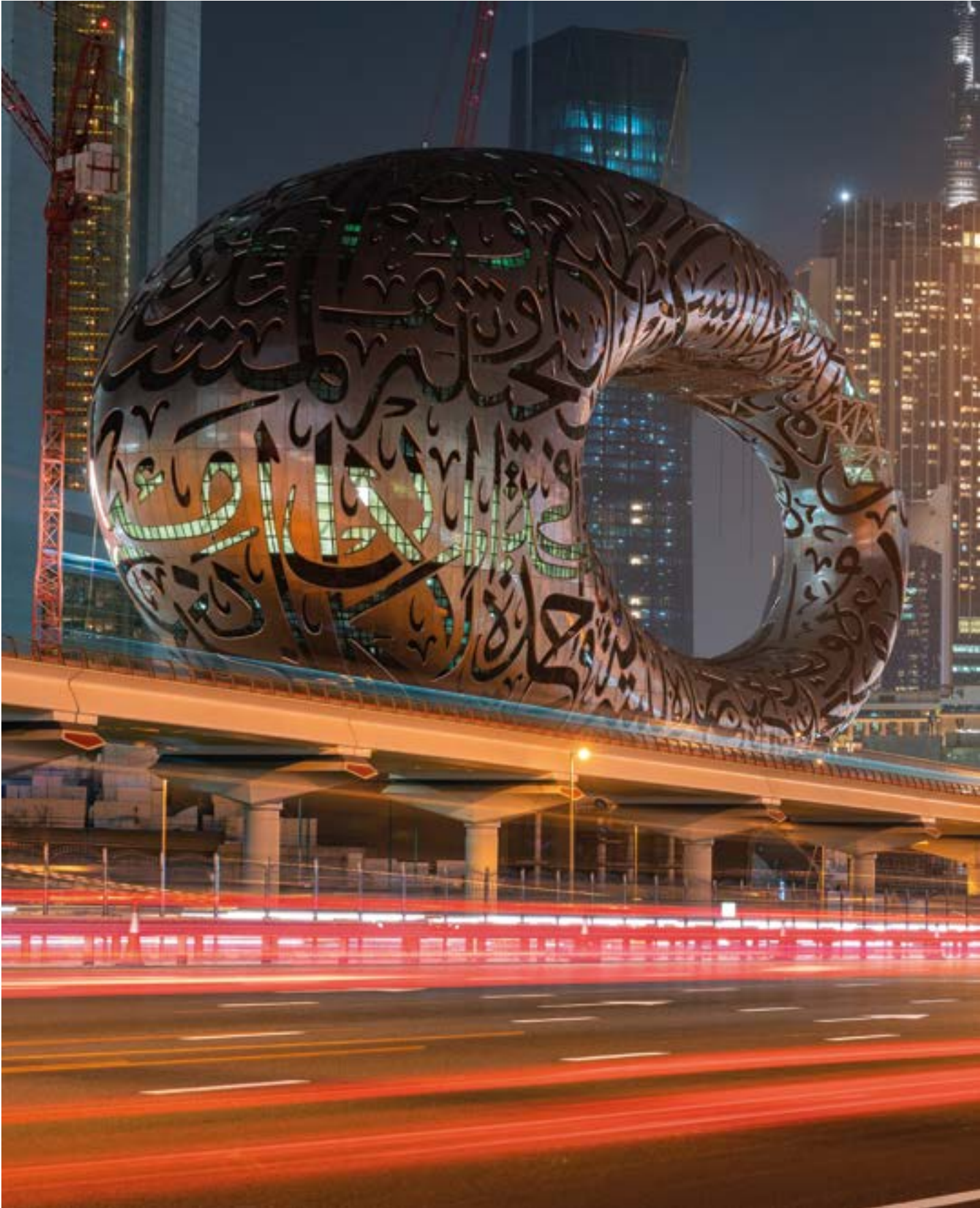
Museum of the future, Dubai (United Arab Emirates) - BAM International
