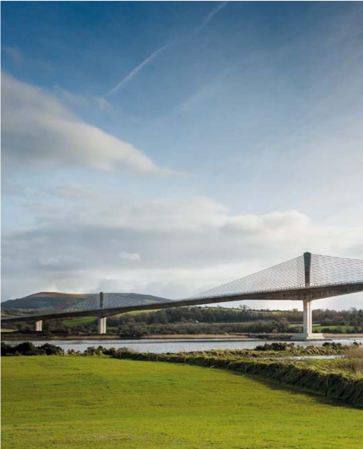
Rose Fitzgerald Kennedy Bridge N25, New Ross (Ireland) - BAM Contractors Ltd and BAM PPP
