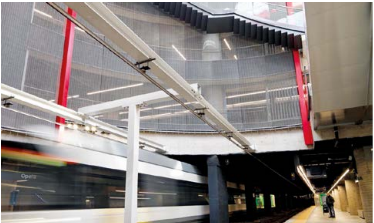
Tramline Brabo 2, Antwerp (Belgium) - BAM PPP and BAM Contractors nv
