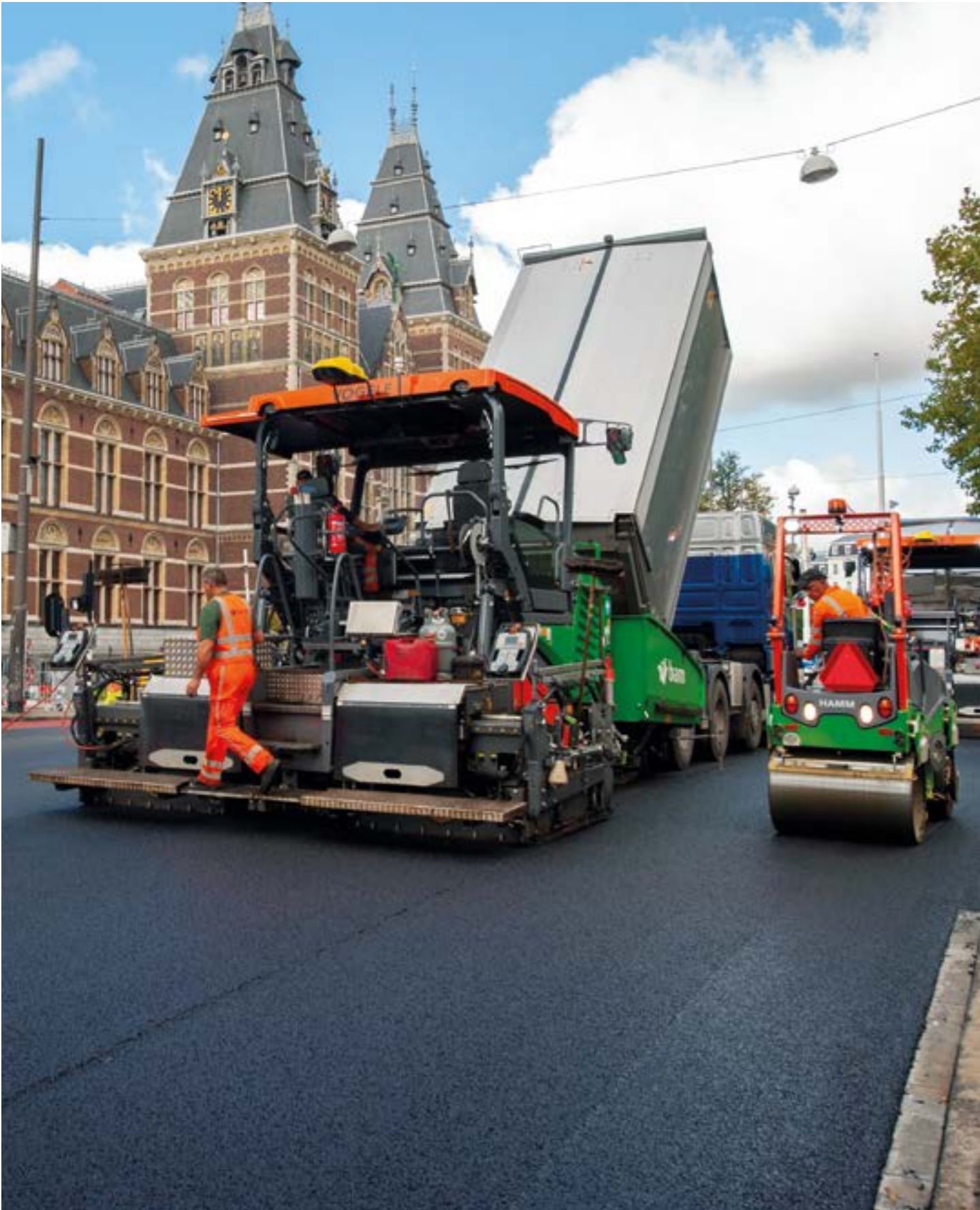
Stadhouderskade Amsterdam (the Netherlands) - BAM Infra Nederland
